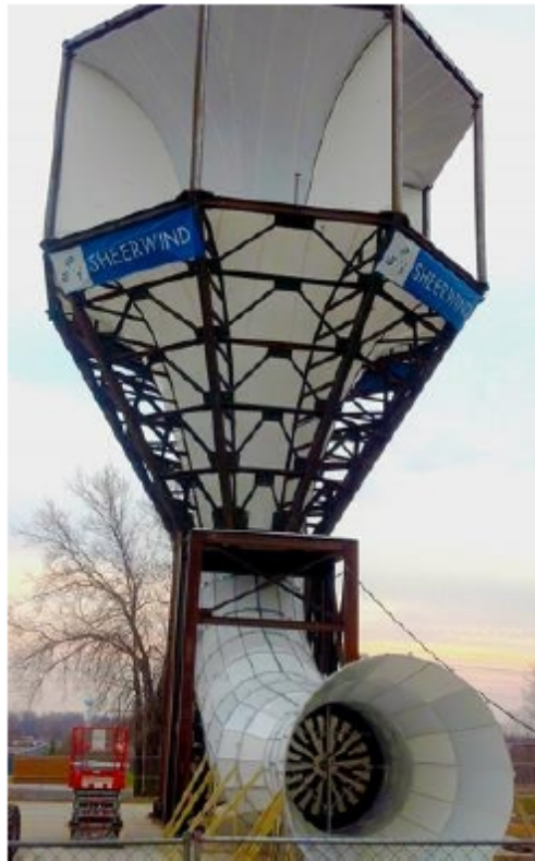
Figure 7: Wind capture and duct concept to accelerate air flow around wind turbines.
