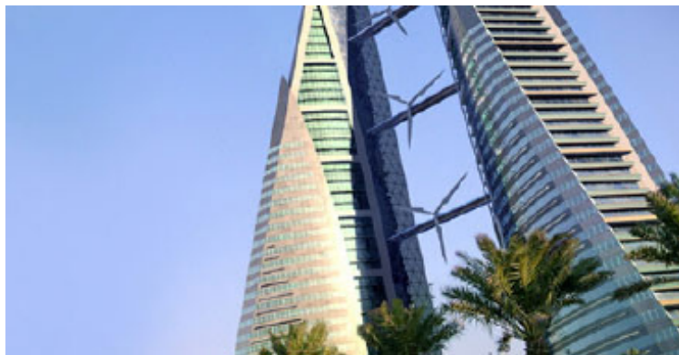
Figure 8: Building design to incorporate wind capture and acceleration to drive wind turbines.
