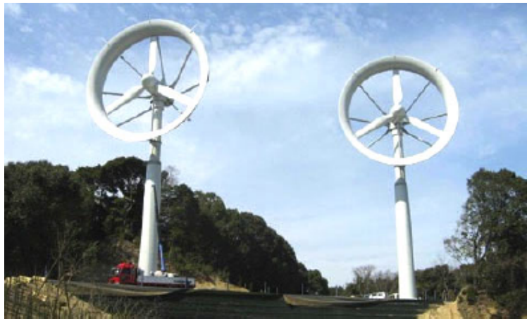
Figure 5: Examples of horizontal wind turbine duct concepts.
