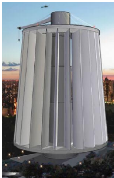
Figure 4: Concept of a giant vertical axis wind turbine mounted on magnetic levitating bearings.
