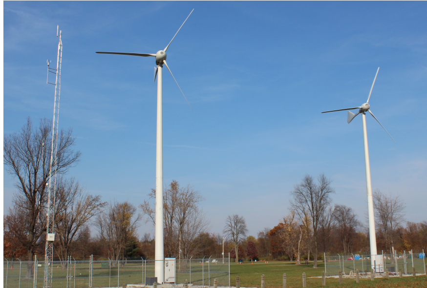
Figure 17: Photograph of the University of Notre Dame Research Wind Turbines and Meteorological tower.
