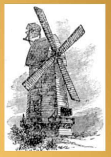
This design incorporated blades attached to a horizontal shaft that used a wooden cog-and-ring gears to translate the motion of the horizontal shaft to a vertical rotation of the grindstone. The miller could manually rotate the post mill into the wind.
