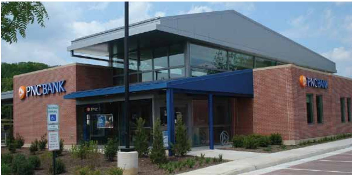
In 2002, PNC became the first major U.S. bank to apply green building standards to all newly constructed or renovated retail branch offices.
