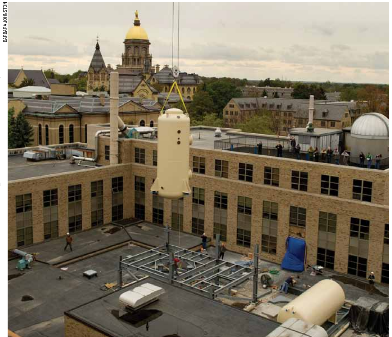
The new particle accelerator, shown here being lifted into position on top of Nieuwland Hall of Science, is 21 feet tall, about eight feet in diameter and weighs nearly 18,000 pounds.
