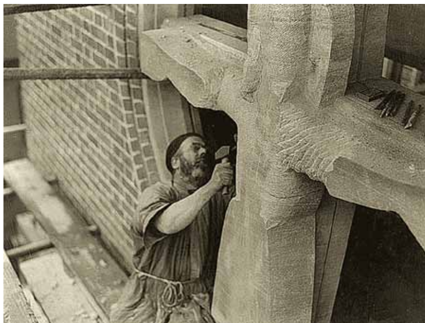
Gill working on the Calvary Group, St. Thomas the Apostle Church, Hanwell, West London, in 1933. The cross was carved from a single block of stone.
