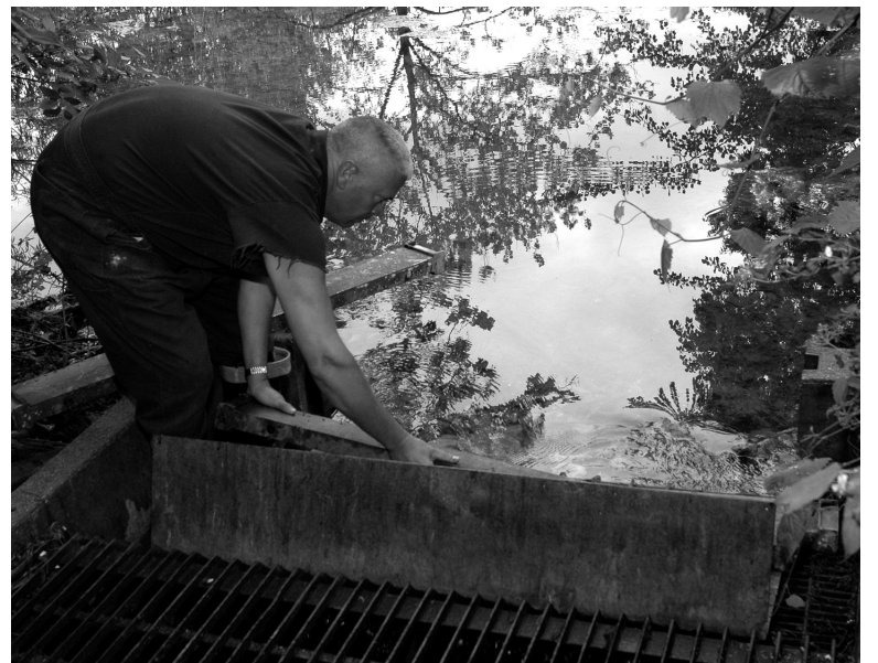
Dan Younggreen of the Utilities Department reinstalls wooden panels that separate St. Mary's Lake from a drain that flows into the St. Joseph River. Before treating an aquatic weed in the lake, its volume was lowered to better retain the treatment substance. Photos by Joe Raymond.
