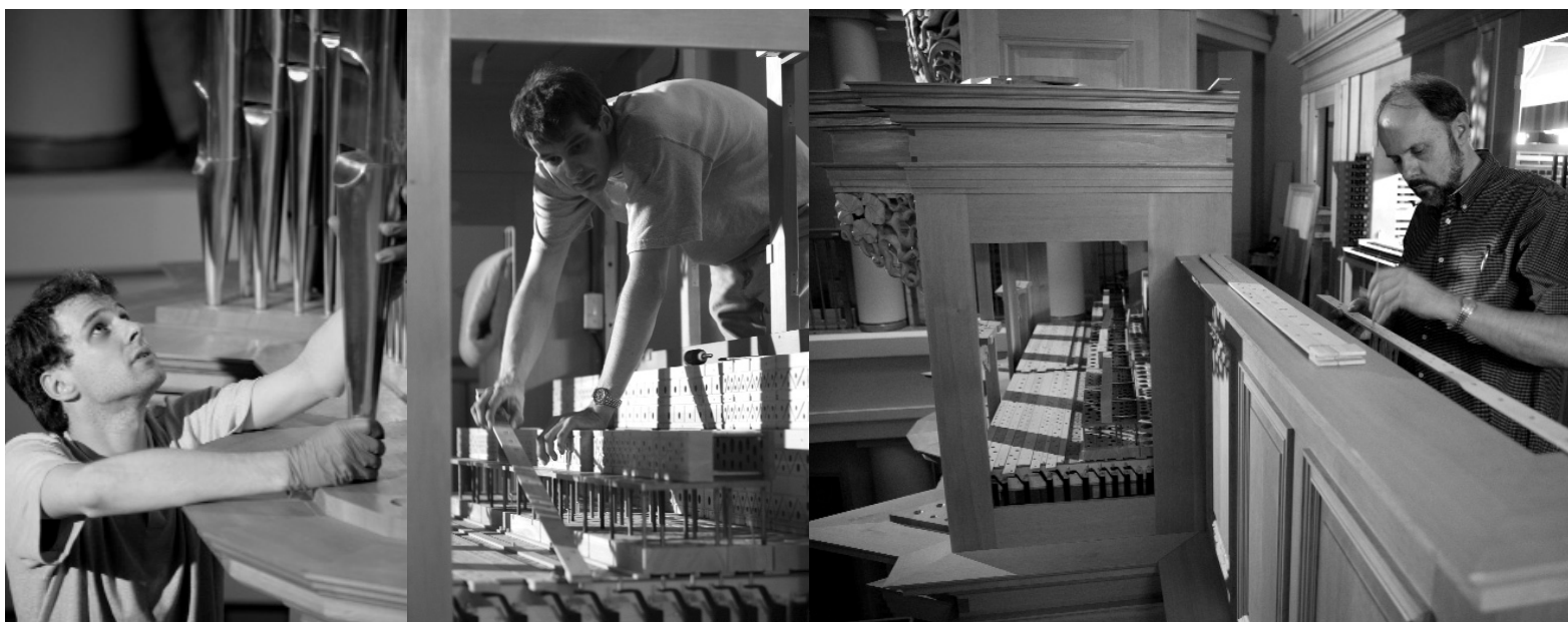
Having assembled the organ in his Washington State workshop, Paul Fritts, right, begins reinstalling it in the Reyes Organ and Choral Hall in early summer. Hand-molded pipes and hand-crafted stops are delicately placed by one of Fritts’ assistants. Photos by Matt Cashore.
