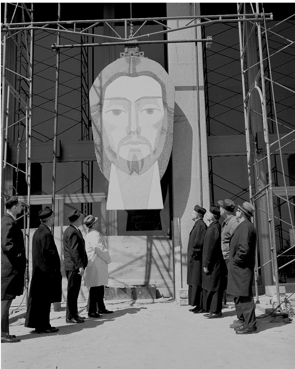
University leaders and supporters gather to see an essential piece of the Word of Life mural put in place. The head of Christ is 9 feet tall and made of 115 different pieces of stone. The library was dedicated May 7, 1964. Photo provided by Charles Lamb, University Archives.
