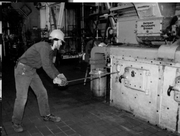
Below: John Murton scrapes ash and residue from the sides of a boiler in the Power Plant. A skeleton crew kept the University functioning over the holiday break.
