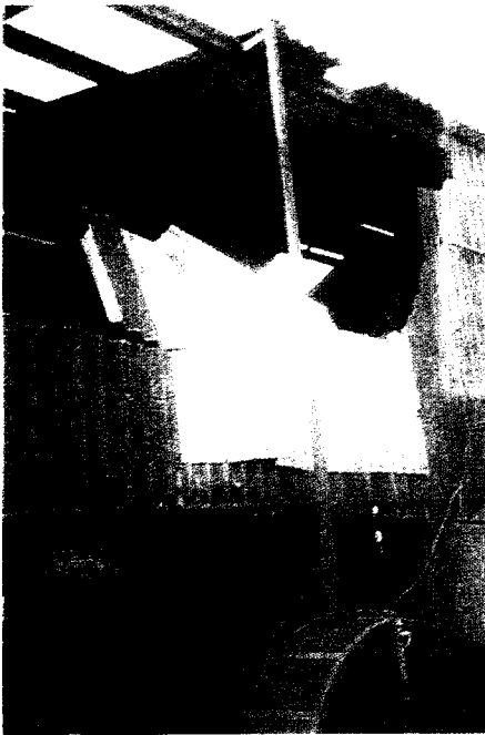
Fig. 21 Typical structural envelope damage analogous to that witnessed on land
