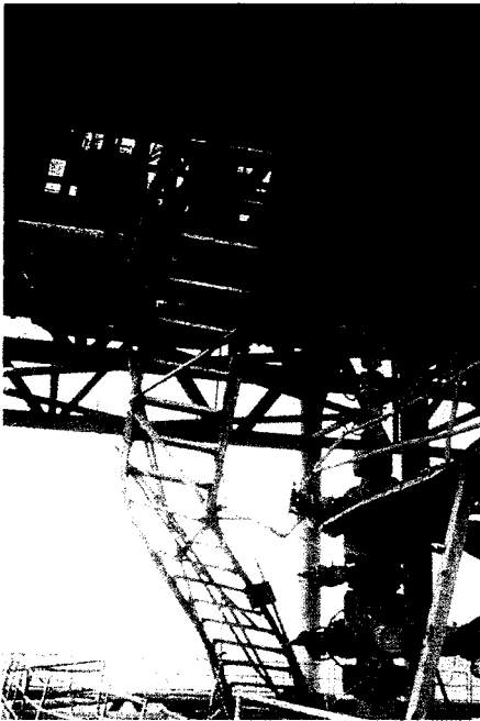
Fig. 18 Damage to deck railing and ladder
