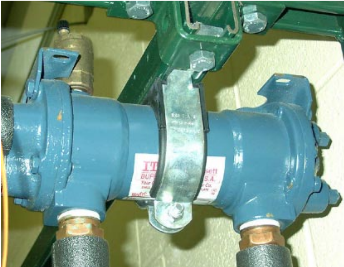
Figure 4.4. Water-water shell-tube heat exchanger.
