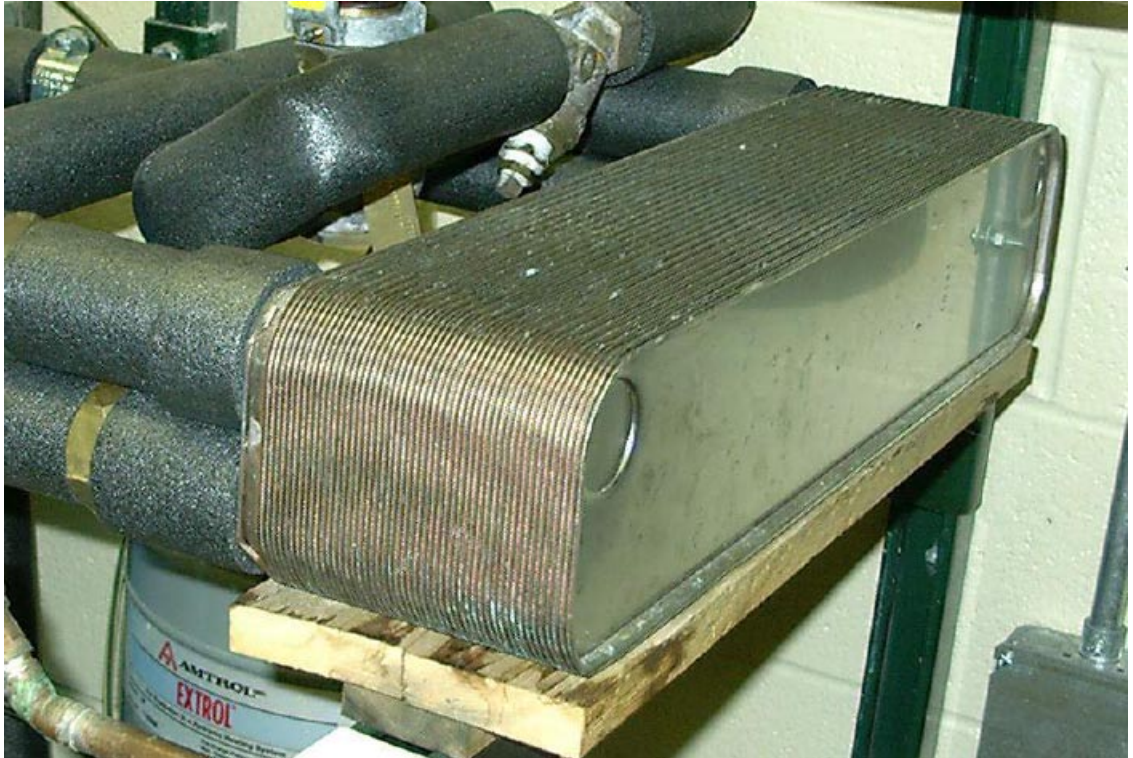
Figure 4.5. Water-water compact heat exchanger.
