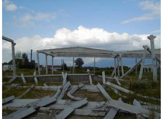
Figure 2 Collapsed industrial building near Adapazarı
