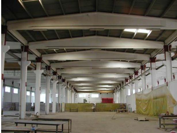
Figure 1 Interior of an industrial building near Düzce
