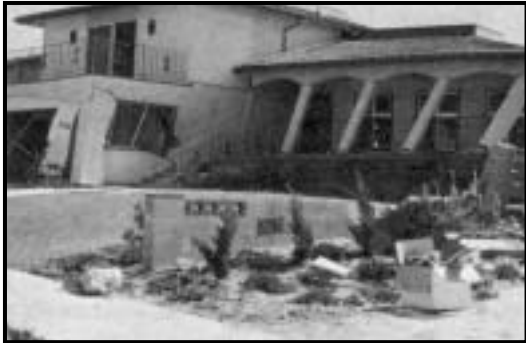
a) Foundation Cripple Wall Collapse
