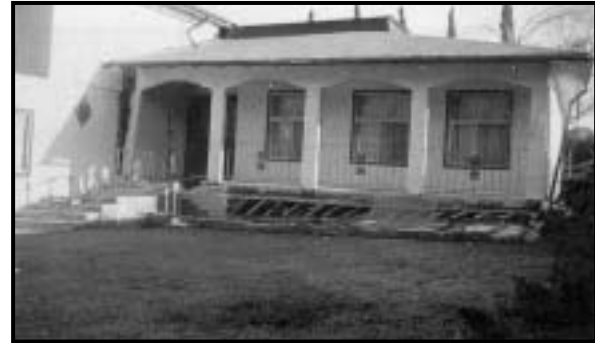
a) Foundation Cripple Wall Collapse
