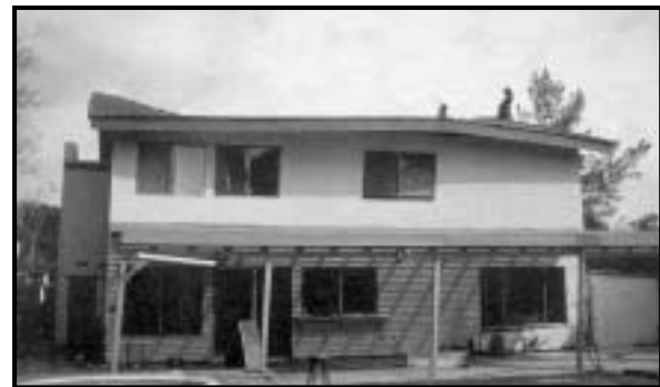
c) Roof Framing Damage
