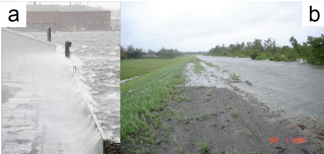
Figure 2: Photographs during Gustav of (a) waves overtopping the IHNC walls near the Ninth Ward, and (b) surge overtopping the earthen levee near Braithwaite, courtesy of Nancy Powell, USACE.
