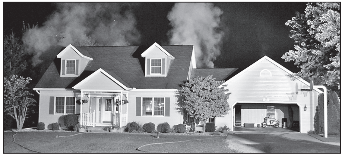
TWO TREATED FOR SMOKE INHALATION ☒ Smoke billows from the east side of the Jeff and Peggy Guyas' residence on CR 450N, Syracuse, early Thursday morning. Two occupants in the structure were treated for smoke inhalation at the scene by Turkey Creek EMS. The fire was ruled electrical in nature with combustible materials stored nearby. (Photo by Deb Patterson)
