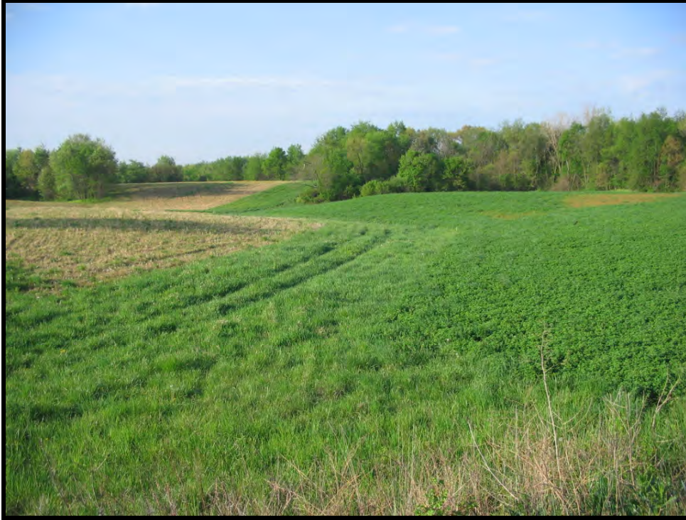
Water and sediment control basin (WASCOB) outlet installed in the Turkey Creek Headwaters through the Watershed Land Treatment Program.
