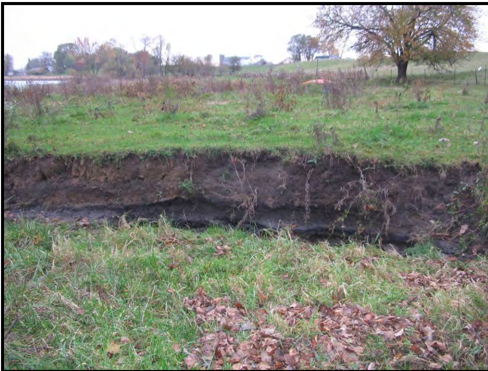
Figure 34. Streambank erosion occurring within a Wawasee Area Watershed stream.
