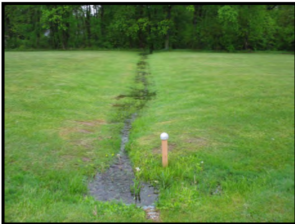
Figure 9.4a. Upstream of road.
