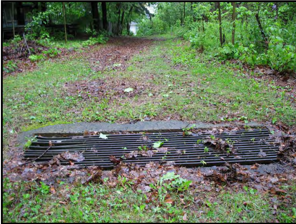
Figure 10.1. Metal grate covering 2x2 foot drain pipes.
