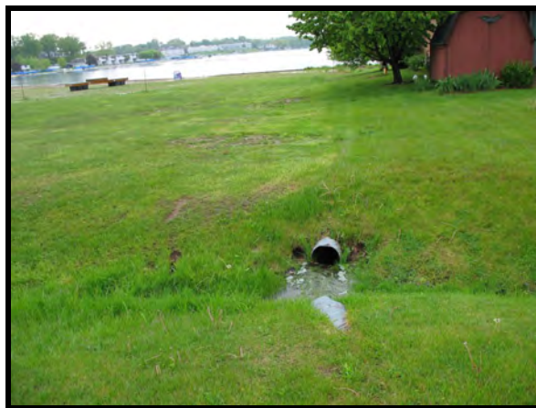
Figure 9.4b. Downstream of road.
